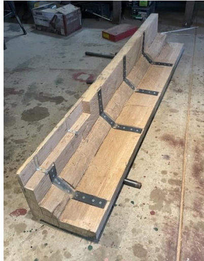
Fig 11. Inside Faux Post to Conceal 21 st C. Mechanicals
