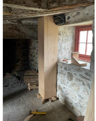
Fig 12. Installing Faux on Wall
