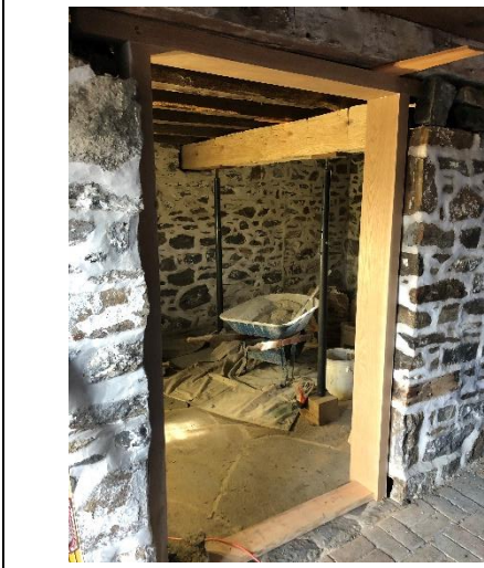
Fig 10. New Beam, Door Frame and Floor
