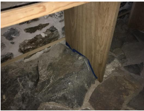
Fig 13. Pantry Feet Scribed to Fit Bedrock Outcropping
