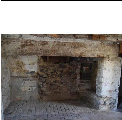
Fig.4. Hearth and Kitchen Floor Restored
