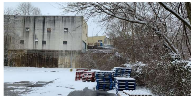
Existing Retaining wall along Caliber Collision
