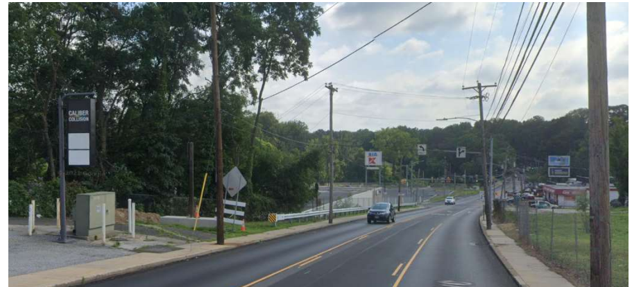
Looking East Along Baltimore Avenue from Western Project Limits in front of Caliber Collision
