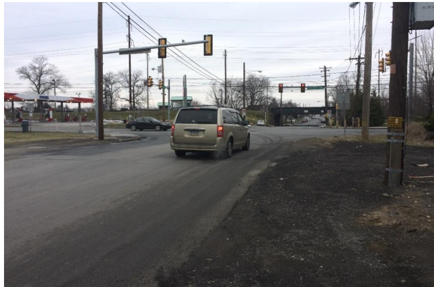
Figure 4-14: PA Route 291 and Saville Avenue, Eddystone Borough
