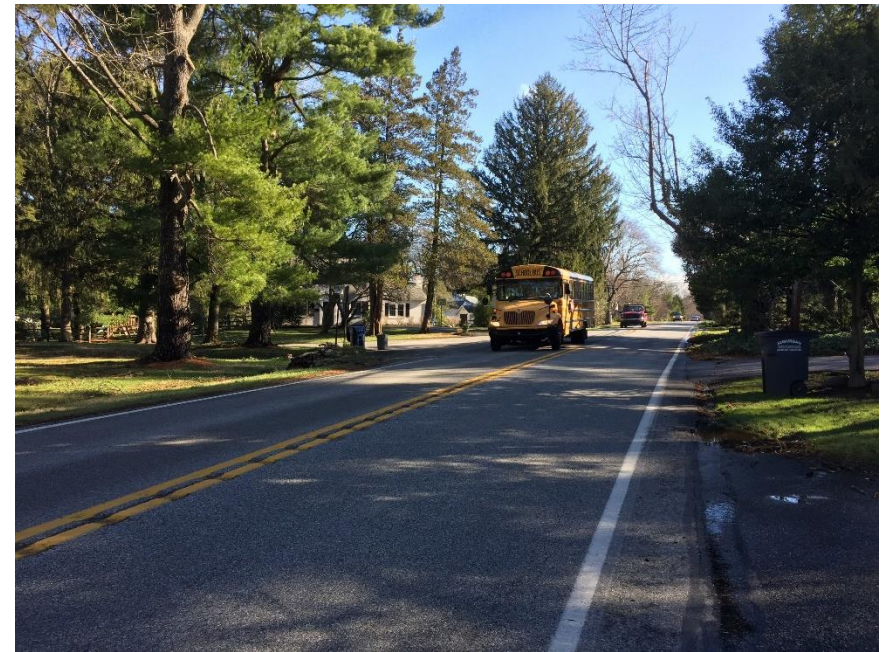
Figure I-2: Nether Providence Township was awarded the Department of Community and Economic Development (DCED) 2017 Multimodal Transportation Fund (MTF) award to construct sidewalks on East Rose Valley Road between Providence Road and Osbourne Lane.
