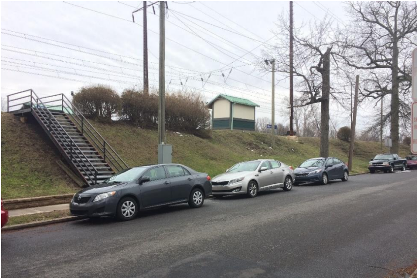
Figure 4-13: Stairway entrance to Eddystone Station outbound platform, Eddystone Borough
