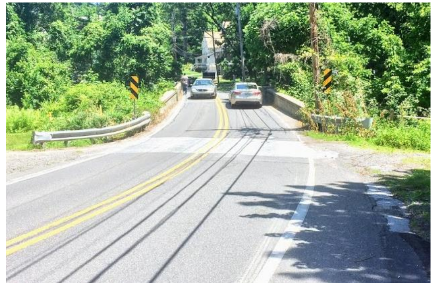
Figure 4-43: Plush Mill Road bridge, Nether Providence Township
