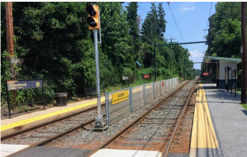
Figure 4-15: Drexelbrook Station, Upper Darby Township
