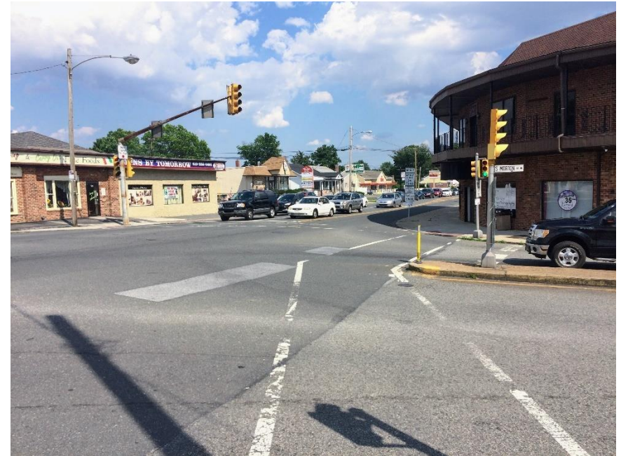
Figure 4-26: PA Route 420 and Morton Avenue, Morton Borough
