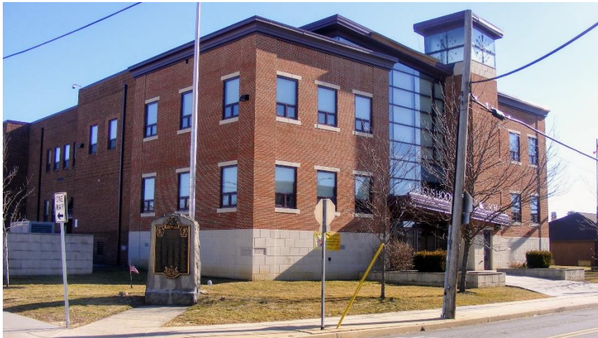
Figure 4-5: Marcus Hook Elementary School, Marcus Hook Borough
