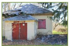
House for the Woodburne Mansion. The 2,200 sq. ft. building, dating from 1907, apparently housed two large generators in its Engine Room, and had a separate Storage Battery Room in the rear. There has been little to no maintenance of this structure for many years. It is not secure, and it is subject to some vandalism. Significant repair work is required, including repairs to the masonry, roof structure, roofing, roof flashings, soffits and trims, and the doors and windows.
