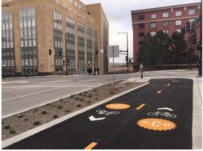
Custom trail Branding graphics can be placed in conjunction with standard paint markings. (Photo credit: armofmn.com)
