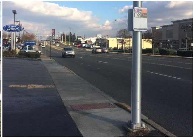
Figure 3-7: This Basic Stop for the 109 Bus along Baltimore Pike has sidewalk access but is lacking passenger amenities.
