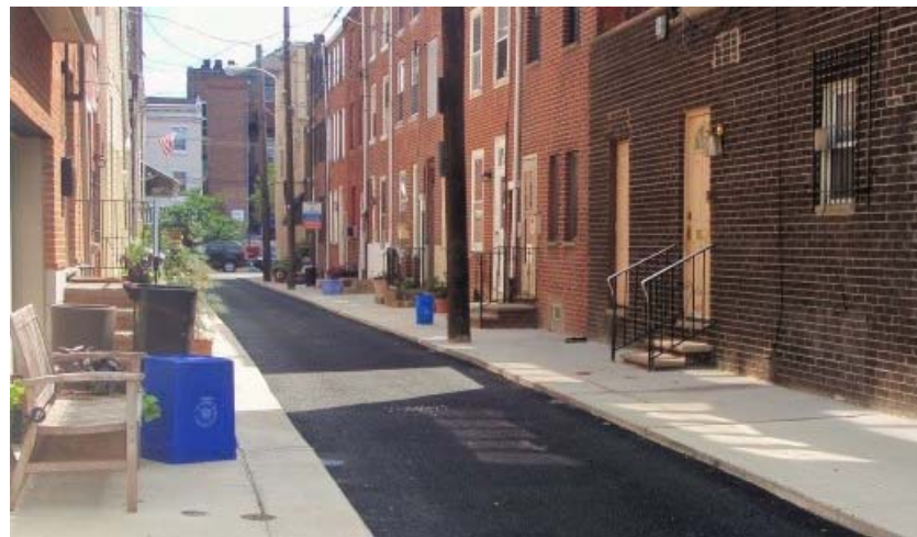
Figure 4-2: The 800 block of Percy Street in Bella Vista is the City of Philadelphia's first porous green street. It is an example of GSI implementation on low impact roadways in dense urban areas, such as those in eastern and southern Delaware County. Source: Philadelphia Water Department
