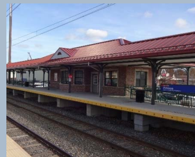
Figure 4-22: Primos Station's high-level platform exemplifies new infrastructure for greater efficiency.
