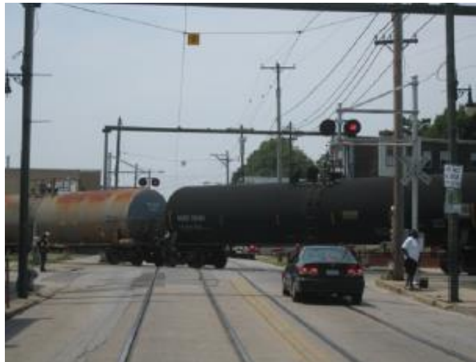
Figure 5-6: The Main Street and 6 th Street grade crossing in Darby Borough is the only grade crossing in the nation where an active freight rail line crosses an active fixed-rail transit line, with vehicular and pedestrian movement through the intersection. The freight rail line is owned and operated by CSX. Source: DVRPC
