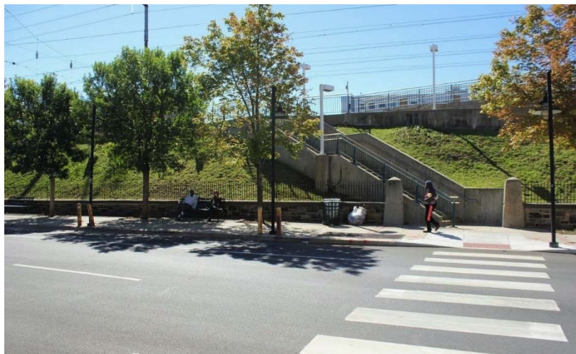
Figure 4-12: In 2016, the City of Chester completed a streetscape project in downtown Chester City. The project included the reconstruction and upgrade of sidewalks, ADA ramps, and crosswalks surrounding the Chester Transportation Center.
